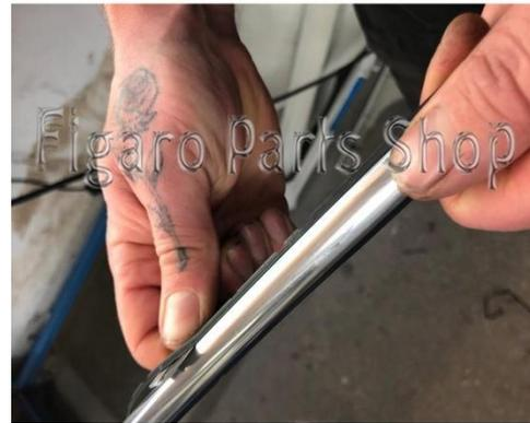
4. You will need to ensure all the old black profile has been removed. This can be done by using the blade to scratch it off the back of the stainless trim or using a combination of heat and a fine sandpaper to achieve this.
